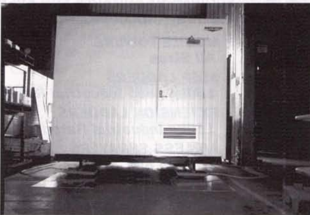
James Hardie Building Systems Ausco transportable washroom 'hovers' into position at SEQEB in Brisbane
