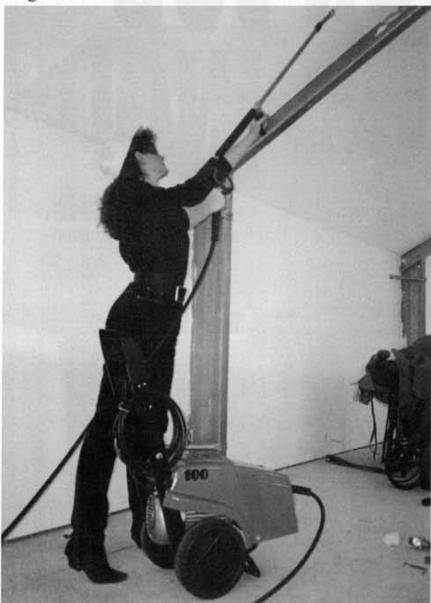
Water blasters can quickly and efficiently clean surfaces which are difficult to reach by conventional methods.
